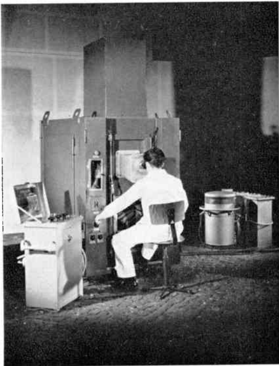
Fig. 5. Special inspection installation used for x-ray examination of cordite.
