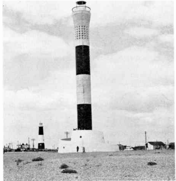
Fig. 5. New Dungeness lighthouse which incorporates electric fog horn and a 2-kW xenon arc discharge light.
