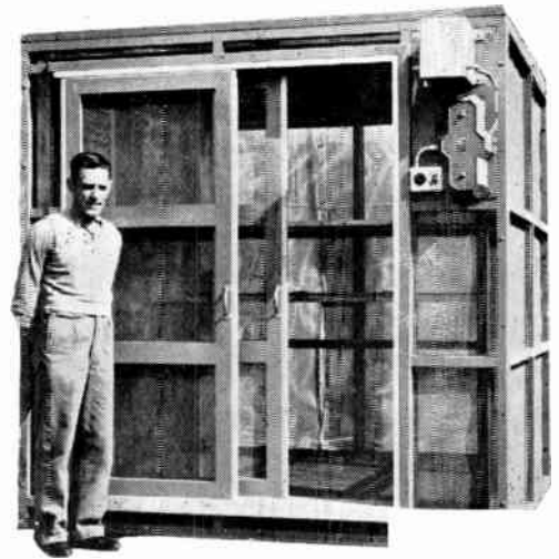
Fig. 3.—Double-screened room with double sliding doors.
