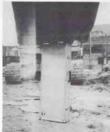
... so we try their digger! No damage.
