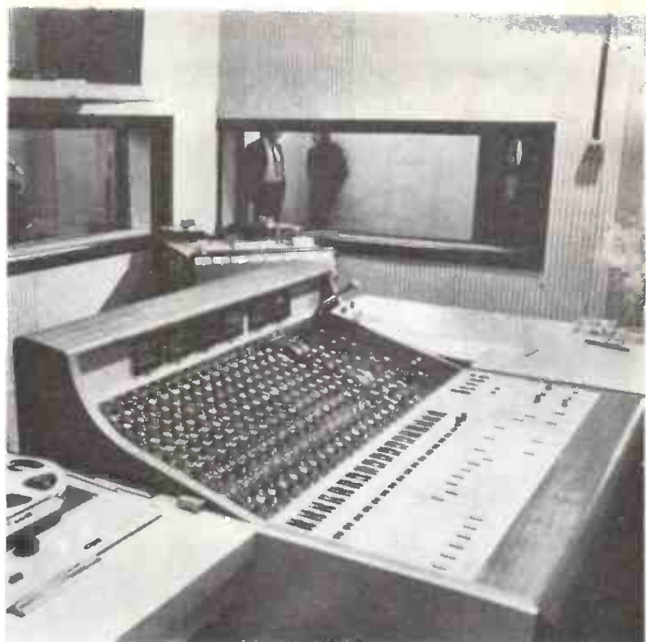
Visual communications with the control room are excellent
