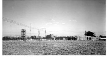
some 2,800 nuts and bolts. The mast base weighed 22 tons and supported a total load of 99 tons when the mast was stayed. In this case there were 9 stays, each set of three being fastened to a concrete base weighing some 64 tons. (Picture above shows the building, feeder runs and switching tower in August 1944)
