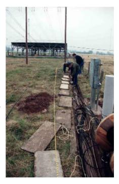
some reason the rodents found the pipes and cable covering edible and they chewed contentedly, eventually causing shut-downs. These manifested themselves when array switches refused to operate, the revertives disappeared or the air compressors supplying the field overheated.
