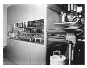
and an even longer time before they were re-installed. Unfortunately many parts of the RF units were missing when the RAF returned them in early spring 1945. In fact S82 ended up with a very modified final RF output circuit, possibly designed by L. F. Ivin. The sophisticated RCA chain driven parallel plate coupling was replaced by a wire lifting up the pivoted output coil, known as the "bedstead".
