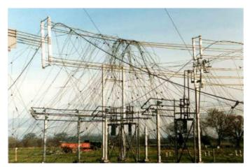
Doodle" spoiling their TV programmes. (Sometimes arcing due to broken dipoles could cause TVI problems if not found. However this storm damage to A953 just before the March schedule change in 1987 was very obvious)
