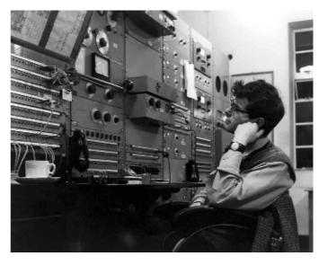
so that LFI could check at any time how his pet mechanism was behaving. This master clock drove all the other operational clocks displayed the building in a series circuit. Senders were switched off and on for the scheduled transmissions by the TAs who used the clocks in each sender hall.
