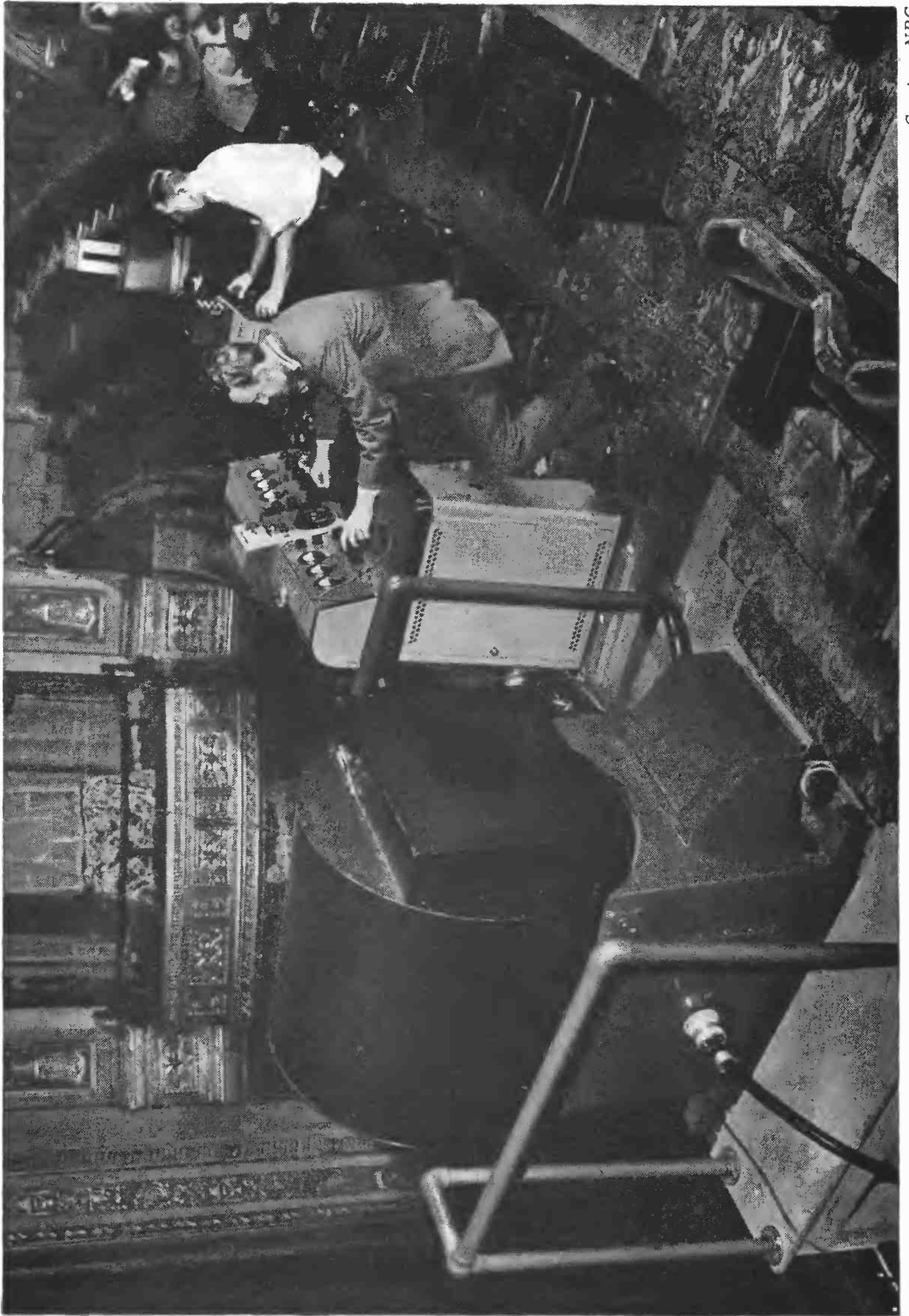
LARGE-SCREEN TELEVISION EQUIPMENT AS INSTALLED IN THE NEW YORKER THEATER
