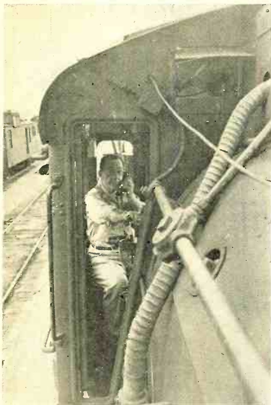
FIG. 5. THE ENGINEER ON NO. 272 CAN GET HIS ORDERS WITHOUT TAKING HIS EYES OFF THE TRACK AHEAD
