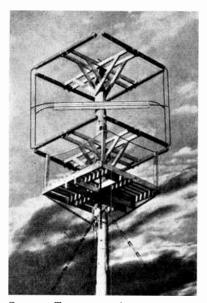
FIG. 1.10D. CUBICAL TELEVISION ANTENNA DESIGNED BY G-E ENGINEERS FOR STATION W2XB Two of these aerials have been erected, one for sound and one for picture transmission. The station is in the Helderberg Mountains in New York State. (Courtesy of the General Electric Co., U.S.A.)
