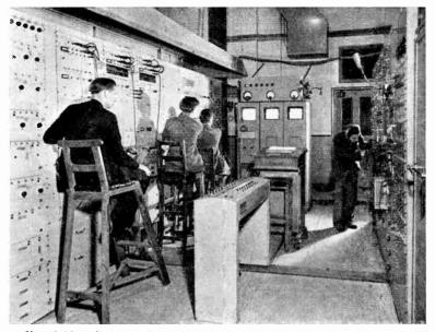
FIG. 1.10B. CONTROL ROOM "A" OF THE B.B.C. TELEVISION STATION Engineers are using the C.R.T. Picture Monitors (centre) to set up the video modulation equipment (left). Audio modulation equipment is mounted in the racks on the right. (Courtesy of the B.B.C.)
