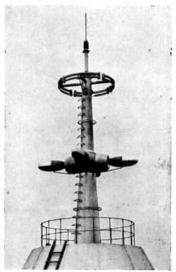
Fig. 169.—Radiator system designed by Lindenblad for station W2XBS, the National Broadcasting Company's transmitter atop the Empire State Building in New York City. The top structure is the folded dipole used for sound transmission, the lower the constant-impedance turnstile structure for the picture signal.
