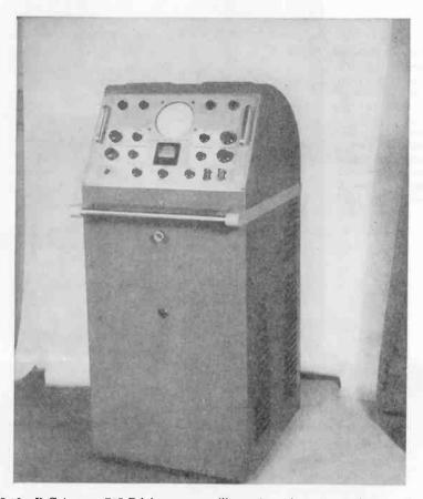
Fig. 3.18 R.C.A. type 715-B laboratory oscillograph, an instrument that may be used at the television control room, at the transmitter, or in the development or research laboratory for routine waveform investigation. It incorporates response which is flat to 11 mc. per sec., triggered sweep, time-base marker (at 1-μ sec. intervals), an input calibration meter, and other features making it especially useful to the television engineer and technician. (Courtesy of Radio Corporation of America.)
