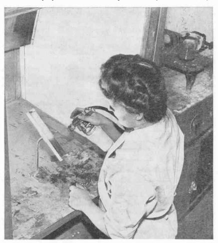
Fig. 2.8 Operator using a spray gun to coat the cathodes of cathode-ray tubes at the Dobbs Ferry, N.Y., plant of the North American Philips Company, Inc. Held in a special platen, 165 of the tiny cylinders have their emissive tips coated simultaneously with the chemicals.
