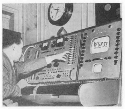
Fig. 11.36 The outputs of the film pickup camera are fed by means of coaxial cable to one or more video input positions at the master control switching and mixing desk. Illustrated is a General Electric master control desk as installed at Station WGN-TV, Chicago. The sound output of the special film projectors is fed to input positions at the master control room audio console. (Courtesy of General Electric Company.)
