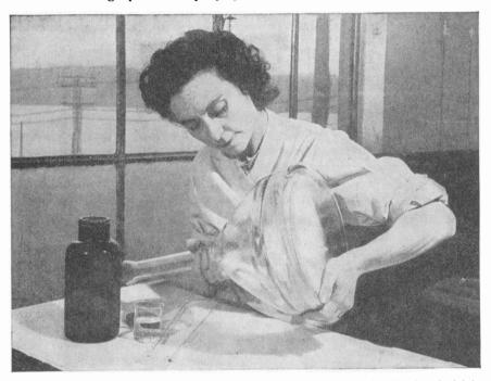
Fig. 2.30 Circular motion applied to a 10-in. cathode-ray tube in the chemical laboratory of North American Philips Company, Inc., at Dobbs Ferry, N.Y. By this method, the phosphorescent powder is distributed over the inner face of the tube. Before the powder is placed in the tube, a liquid adhesive is applied to the inner surface. This makes the phosphor adhere permanently to the glass. (Courtesy of North American Philips Company, Inc.)
