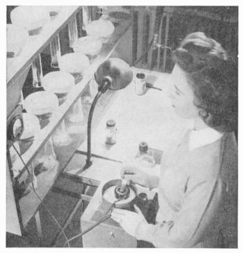
Fig. 2.31 Spectral apparatus for measuring the thickness of the phosphorescent coating which has been applied to the face of the tube. (Courtesy of North American Philips Company, Inc.)
