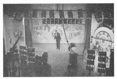
Fig. 1.4 Incandescent-lighting installation in use in Studio A, Station WABD, New York. Iconoscope cameras are being employed. They were later replaced with studio-type Image Orthicon cameras. (Courtesy of Du Mont Television Network.)
