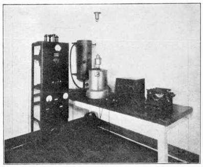
FIG. 155b.—Two-kw. Federal Arc transmitter.
