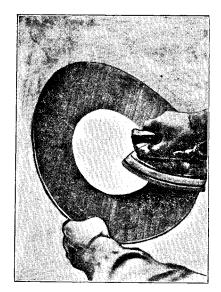
FIG. 3-A repair kink for that busted speaker-cone.
