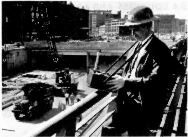
Figure 5-6. Another example of the sound-level meter in use: measuring noise level at a construction site.
