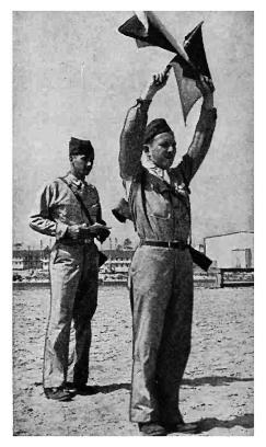
FIG. 1-4.—Sending a message by semaphore. (From the Special U.S. Army Signal Corps Issue of Radio News, photograph by U.S. Army Signal Corps.)
