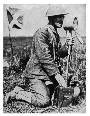
FIG. 1-5.—Signaling by means of a heliograph. (From the Special U.S. Army Signal Corps Issue of Radio News, photograph by U.S. Army Signal Corps.)
