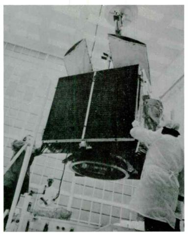
Fig. 11-1. RCA's Satcom IV is prepared for launch at Cape Kennedy, Florida (courtesy RCA Government Systems Divison).
