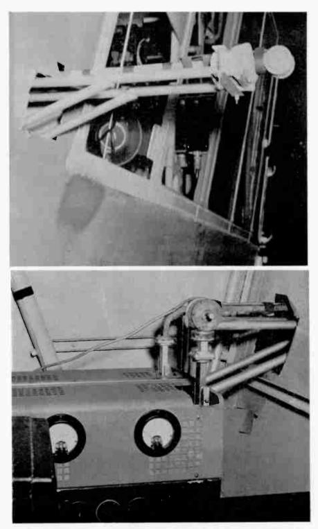
FIG. 1. Composite interior and exterior views of first airborne refractometer installation on a U.S. Navy blimp in 1951. The perforations in the Crain refractometer cavity are those which were used in all future flight programs for ventilation purposes.
