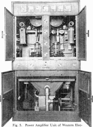
Fig. 5. Power Amplifier Unit of Western Electric 5-KW Radio Transmitter. Front View with Door Open Courtesy of Western Electric Company, New York, N. Y.
