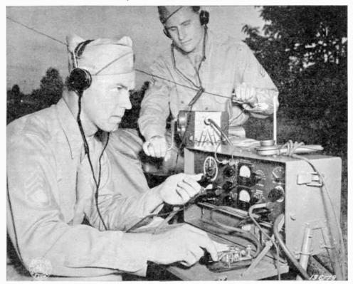
Radio Transmitter in Use in the Field. Man at Right Is Operating the Generator Official Photograph, U. S. Army Signal Corps
