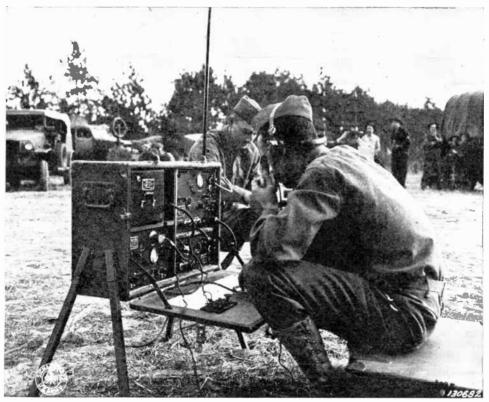
Portable Transmitter and Receiver which Can Be Operated with Phone and Key Official Photograph, U. S. Army Signal Corps
