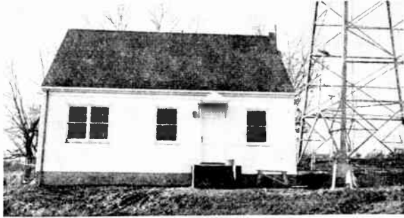
Fig. 3—Transmitter Building (front view).
