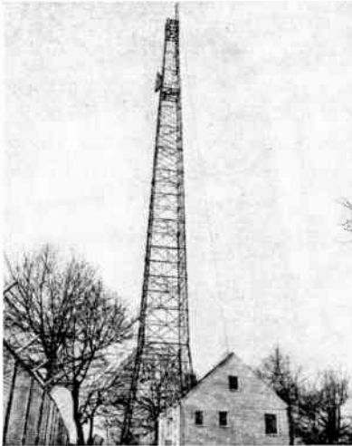
Fig. 6—Transmitter building (side view) and antenna tower. The Channel 4 parabolic receiving antenna can be seen at the 160 foot level of the tower.
