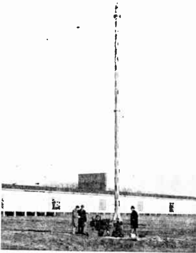
Fig. 2—Antenna installed in the normal vertical position in a rotating socket for measuring horizontal patterns.
