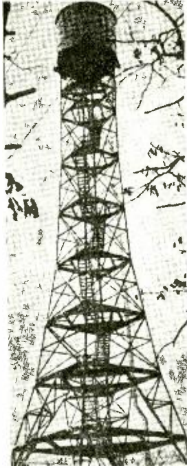
Fig. 3—Hauppauge tower and penthouse.
