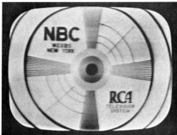
Figure 58—Loss of High Video Frequencies
