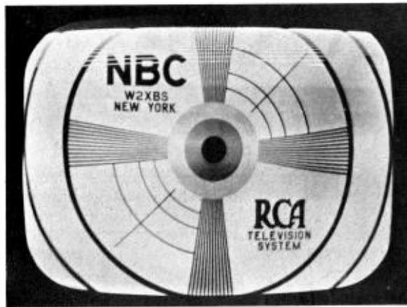
**Figure 55—Vertical Distortion Caused By Defective Peaking**
