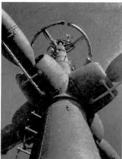
Left — The appearance of NBC's futuristically designed television antenna atop the Empire State Tower in New York was changed in the Fall of 1945 by the addition of new structure (right) to enable field tests of a new RCA 288-megacycle video transmitter. Below— The new high-frequency transmitter.
