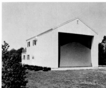
Fig. 1—Antenna development facility at Deptford. The curved radio-transparent wall used for "indoor" testing of antennas is at this end of the building.
