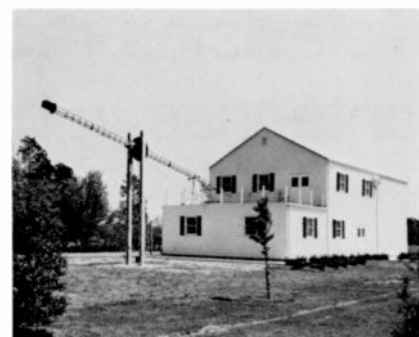
Fig. 2—This end of the antenna development facility shows the tower at one end of the radiation-pattern measurement range.
