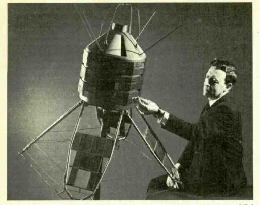
J. B. Atkinson of G.E.C.-A.E.I. (Electronics) Ltd. seen with a half-size model of U.K.-4. G.E.C.-A.E.I. will be producing a good deal of the electronic equipment for the satellite.
