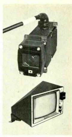
The photographs show a television camera and monitor, produced by E.M.I., that will be used on the Concorde prototype 002 which is due to make its maiden flight from Filton, Bristol, shortly. The camera incorporates printed scan-coils and a 26mm vidicon tube. The monitor employs a 230mm (9 inch) tube and has been designed so that it may be rapidly positioned in front of the pilot should the nose of the aircraft fail to droop during the landing procedure.
