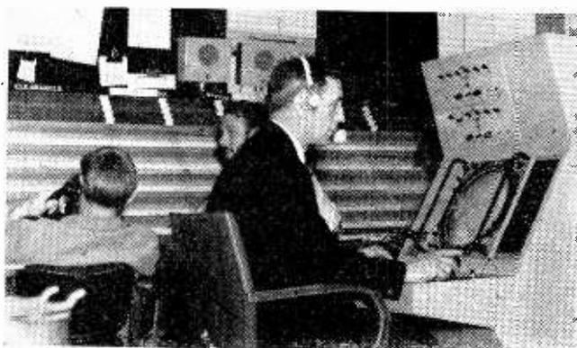
Marconi S264 long-range and terminal area surveillance radar system at Jersey Airport.
