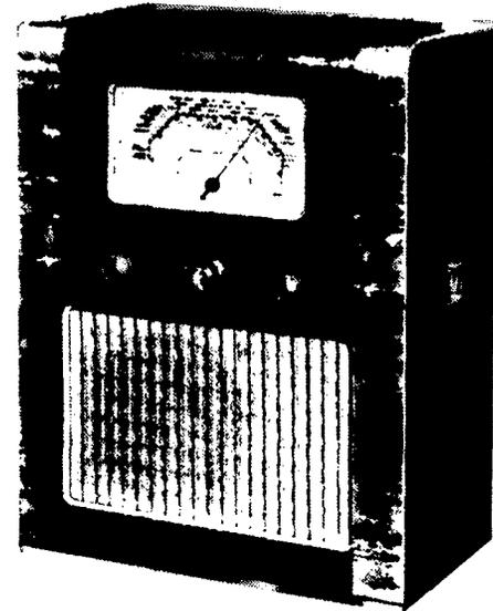
Cossor Model 31 all-wave 4-valve battery receiver.
