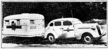
MOBILE STATION. The latest unit of the United Broadcasting Company of America which comprises a trailer studio and a transmitter in the car. It operates in conjunction with WHK, Cleveland, Ohio, and its associated stations WCLE, WHXC and WXBN.
