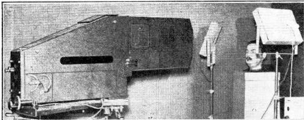
The Baird 30-line Spot-light scanner which was used in the B.B.C. transmissions up to 1932. The banks of photo-cells can be seen on either side of the head.
