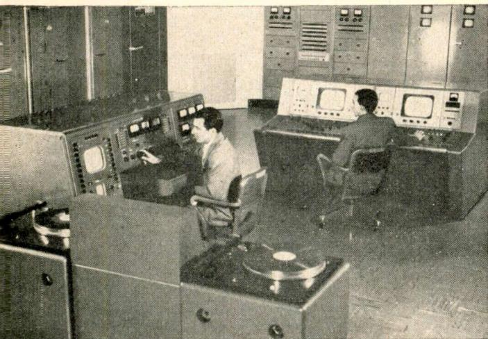
WOR TV engineers Frank Garufy and James Long (l. to r.) operate TV signal in the transmitter building. Foreground equipment is "sound desk" for playing records. Cabinets in background hold reserve transmitter equipment for replacements and emergencies
