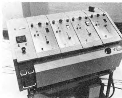
**The new BBC sound effects console, showing a loose cassette at the top right. This unit is built up of four, interchangeable modules**
