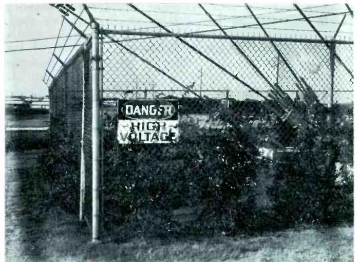
Fences like these around guy anchors will aid in preventing damage. Note the use of the "Danger-High Voltage" sign.
