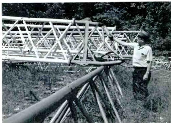
Stacked pieces of damaged tower. Cut guy wire was responsible for damage shown here.
