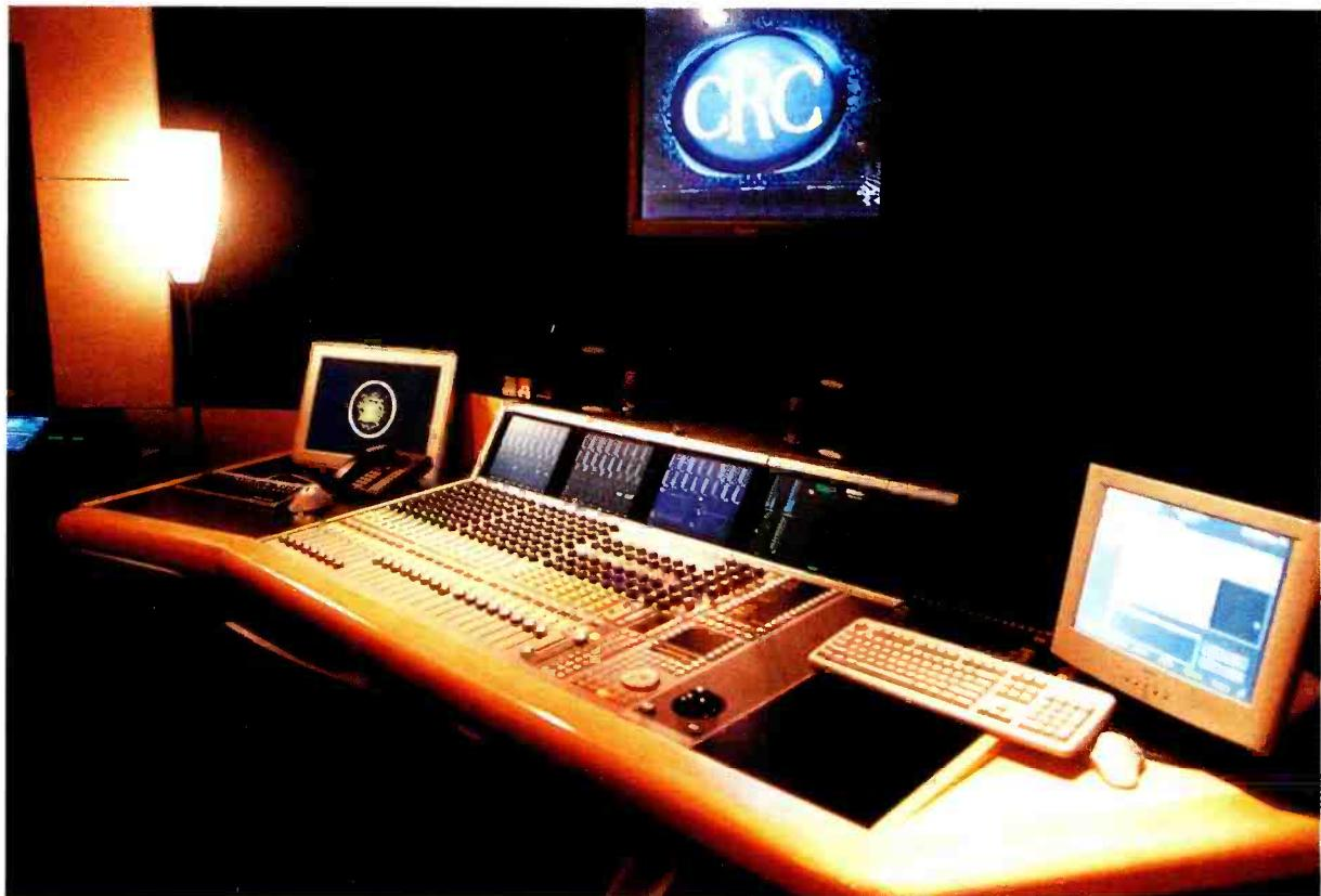
**US:** Mark Ruff's 15 years at the Chicago Recording Co have recently been rewarded by the complete refurbishment of his production studio facilities. The newly-installed Euphonix System 5 console is Chicago's first, and is paired with a Pro Tools system and 5.1 monitoring to provide greater flexibility for Ruff's work in mixing and producing broadcast television and radio spots for US ad agencies. Recent assignments include spots for Miller Beer and AT&T.
