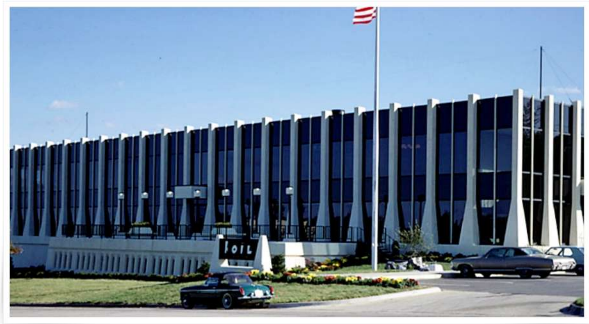
KOIL AM and FM new building near 90th and Dodge Streets 1968. The two poles on top support a long wire for the auxiliary transmitter, KOIL's old 1000 watt RCA transmitter from the 1930s now housed at the studio site for backup. (Courtesy: Deane Johnson collection).
