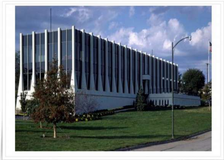
KOIL Building, view from its northeast corner, 1968.
