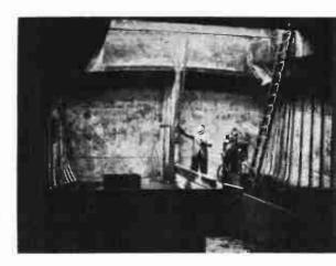
The hold is prepared for the addition of 200 tons of concrete as ballast.
