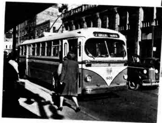
Numbered among recent civic improvements are the new Trolley Buses which now provide efficient and speedy transportation for the Dominion's fourth largest city!
