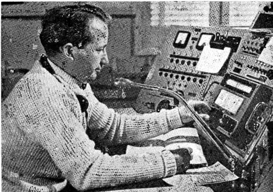
Not, as you may think, rather a fine amateur station with the operator tuning in DX — but the control console at GLD, Land's End Radio, the famous Post Office coast station, equipped to work ships on MF, HF and VHF, using the most modern apparatus and handling a great deal of traffic. Like several other coast-wise G.P.O. stations, GLD functions on what is known as the short-range service, working to craft of all nationalities in the approaches to the English Channel and the Irish Sea.
