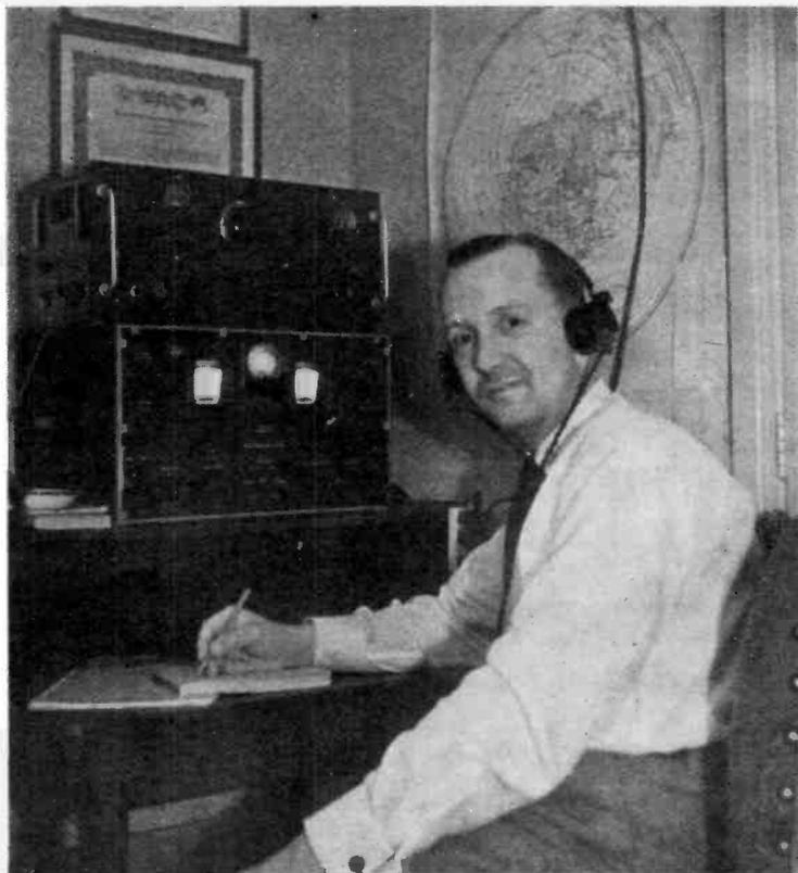
PA0VD, Rotterdam, is ex-PK4VD (1947-'48) and now has a neat living-room layout running, as he says, "moderate power." The transmitter is EF50-EF50-6V6-807, covering 3.5, 7 and 14 mc, but operated mainly on 40-metre CW; the power supply is on the same chassis as the transmitter, the whole of this part of the assembly being in a BC-348 cabinet. Receiver is an HQ-120 and the aerial a 7 mc doublet. Some 55C have been worked post-war on Forty.
