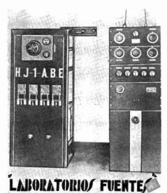
HJ1ABE "Laboratorios Fuentes", Cartagena: Above—the new transmitter recently installed in Cartagena and now working on 6115 kc. or 49.05 meters, under the title "The Voice of the Fuentes Laboratories." The station is rated at 160-180 watts power, and provides reception throughout the world. The special "DX" tests, transmitted each Monday, from 10:30-11:30 p.m., transmitted each Monday, from 10:30-11:30 p.m., wave "fans."
