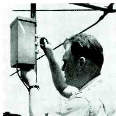
**INSTALLING** a mast-mounted preamplifier.
