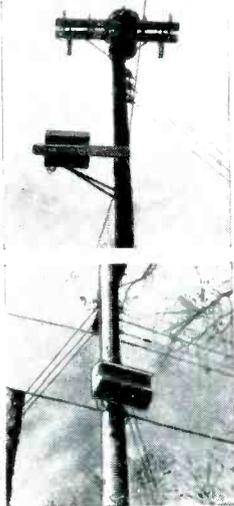
Two views of SKL Model 212TV Amplifier mounted in Model 420 Amplifier Cabinet, mounted on a telephone pole crossarm (top), pole (bottom). Courtesy Vermont Television, Inc.
