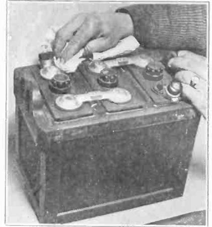
FIG. 6—The storage battery must be kept free from corrosion. A battery whose terminals are covered with corrosion, is a battery whose life will be comparatively short. Keep the battery clean and you will be rewarded with long, care-free service.
