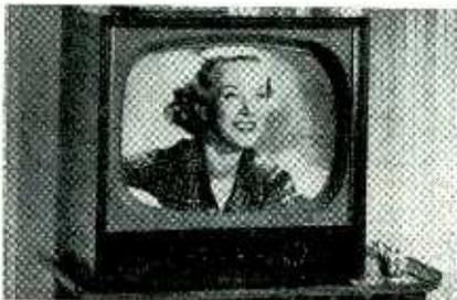
105, the new chassis is designed especially for long distance reception. It employs 21 tubes, including two rectifiers and the picture tube. Magnavox Company, Fort Wayne, Ind.—RADIO & TELEVISION RETAILING.
