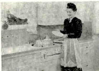
the dual operation of spraying the dishes clean and spinning the basket in which they are carried. Available in deluxe model, embodying a hydraulic lift which, with the turn of a knob, raises the basket out of the finished aluminum basin. The standard model lacks this hydraulic lift. Both models are furnished either in a white, enameled cabinet or a chassis to be built into the sink cabinet of the home. Kaiser Fleetwings, Inc., Kaiser Bldg., Oakland, Calif.—RADIO & Television RETAILING.
