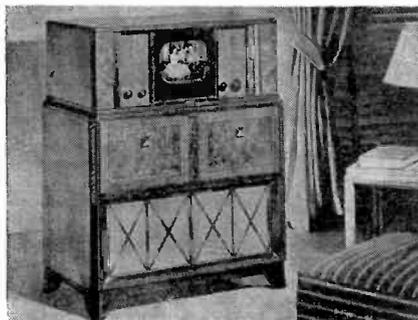
nels. Ten-watt output push-pull amplifier, four positions of tone control. Single external tele antenna also works for FM, shortwave and standard. Four rectifiers, plus 36 other tubes, plus picture tube. Period design cabinets in walnut, mahogany or blonde mahogany. Measures 33 1/4" wide by 46" high by 21 1/2" deep. \$795 exclusive of tax and owner's policy fee of \$79. RCA Victor Division, Radio Corp. of America, Camden, N. J.—RADIO & Television RETAILING.
