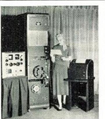
COVER PHOTO: CGS Laboratories' unique "Trak" code converter which "translates" code into English copy at high speed. The unit also incorporates "memory" circuits which will store up to ten textual characters. (Ektachrome by Hugh Stern)
