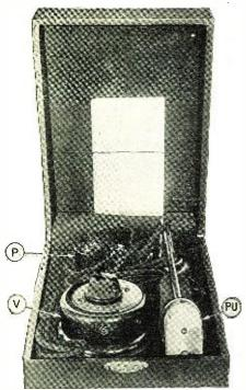
The parts of the "recreator" as they appear in their carrying case. PU, magnetic pick-up; V, volume control; P, plug.
