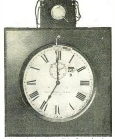
Above, the face of the Time Chime just befor the signal; the minute hand has closed a switch, A, as shown in the diagram below. Twelve seconds before the signal, the second hand closes another and the pilot lamp. L, lights. The announcement is then made to the radio audience, and the Western Union signal strikes the chime, which goes out through WRNY's transmitter.
