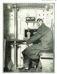
HE motor equipment here illustrated was built for the use of the British post office, which has jurisdiction over radio, as well as all telephone and telegraph service in the United Kingdom; and is now being utilized to detect oscillating sets, which are prohibited by law.
