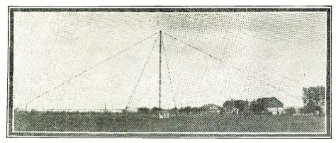
The radio beacon at Wilbur Wright Field, showing the directional triangular loop.
