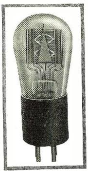
The "Quadrotron" tube. The triangular object mounted in the center of the assembly constitutes the fourth element or "control grid."
