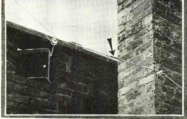
placed at least two feet apart. The lead-in should be taken from the exact middle of the antenna.
