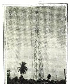
A typical steel construction radio tower. All members are galvanized to protect them from deterioration through climatic influences. Photo courtesy of Milliken Brothers Mfg. Co.
