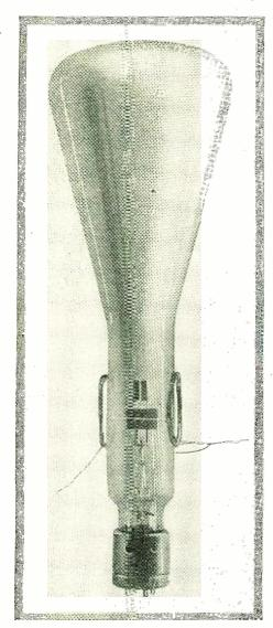
A commercial form of eathode oscillograph with coils attached for obtaining characteristic curves of vacuum tubes.
