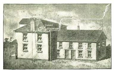
ty, Ontario. The main part of the lightning stroke left the aerial and passed down through the house, resulting in almost com-plete destruction of the front part of the building. The damage is estimated at about \$7,000.00.
