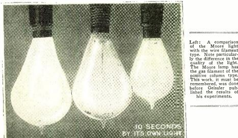
Left: A comparison of the Moore light with the wire filament type. Note particular-ly the difference in the quality of the light. The Moore lamp has the gas filament of the positive column type. This work, it must be remembered, was done before Geissler pub-lished the results of his experiments. his experiments.
