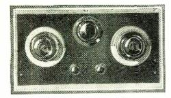
ront panel view showing exceptionally sym-etrical arrangement of controls. All actual tuning is done with the two vernier dials.
