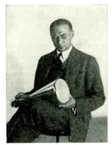
This bottle-like object is a cathode ray tube which forms the receiver of the new type of television invented by Dr. Zworykin, who is holding it. The broadcast pictures appear on the round end of the tube and from there are projected on a mirror in view of the spectators.
