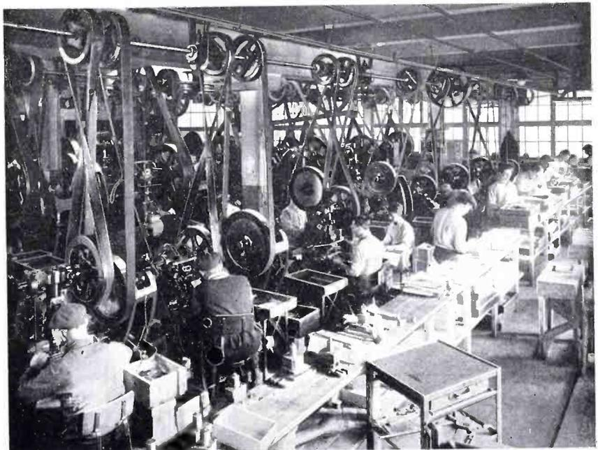
Fig. 2. A part of the stamping department, where holes are punched and special shapes stamped into the panels
