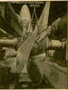
Westinghouse Photos Propeller is shaped by large cutting burrs.
