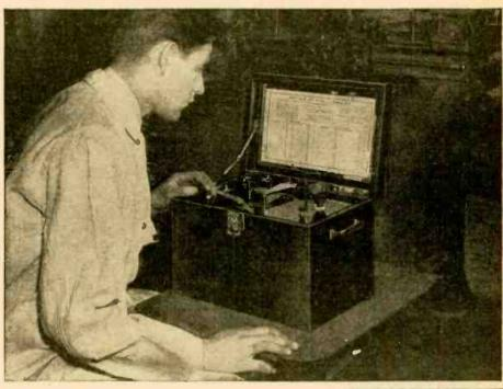
TIME-SAVING carbon content analyses of steel samples-from molten metal to report-take only five minutes with the portable, battery-powered Carbanalyzer, produced by the Fisher Scientific Company. Leading steel firms employing open hearth or electric furnaces quickly make carbon determinations of each batch, achieving close control of quality.
