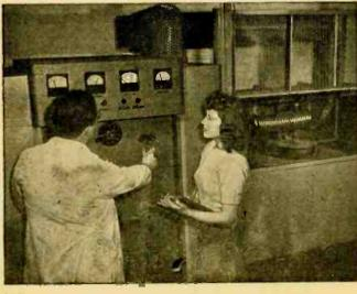
Checking adjustments on the high-frequency rubber vulcanizer. A small tire, seen under the disc-shaped plate at right, is un dergoing treatment. Note the shielding screen around work and directly above the apparatus.
